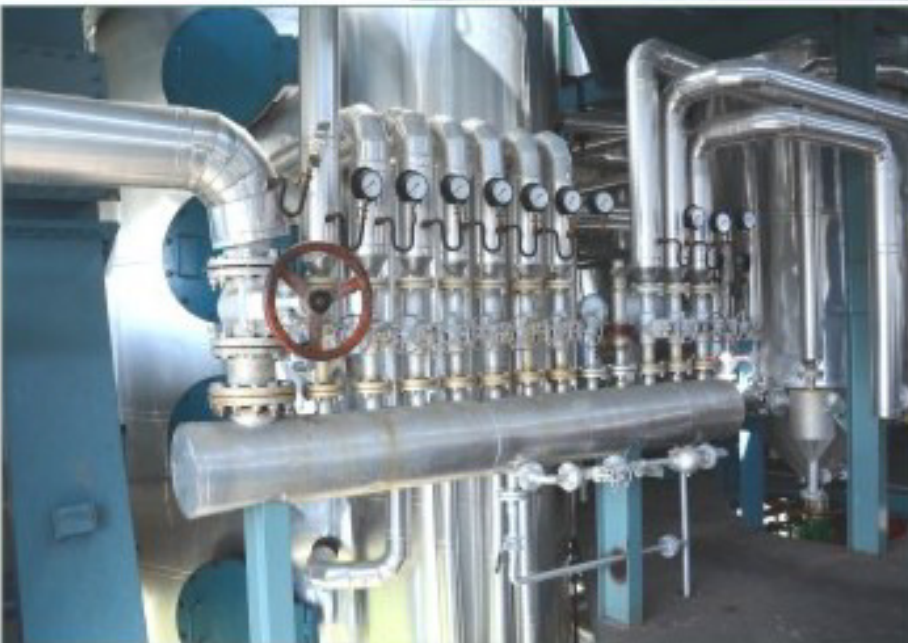
View of Steam Header Solvent Extraction Plant
