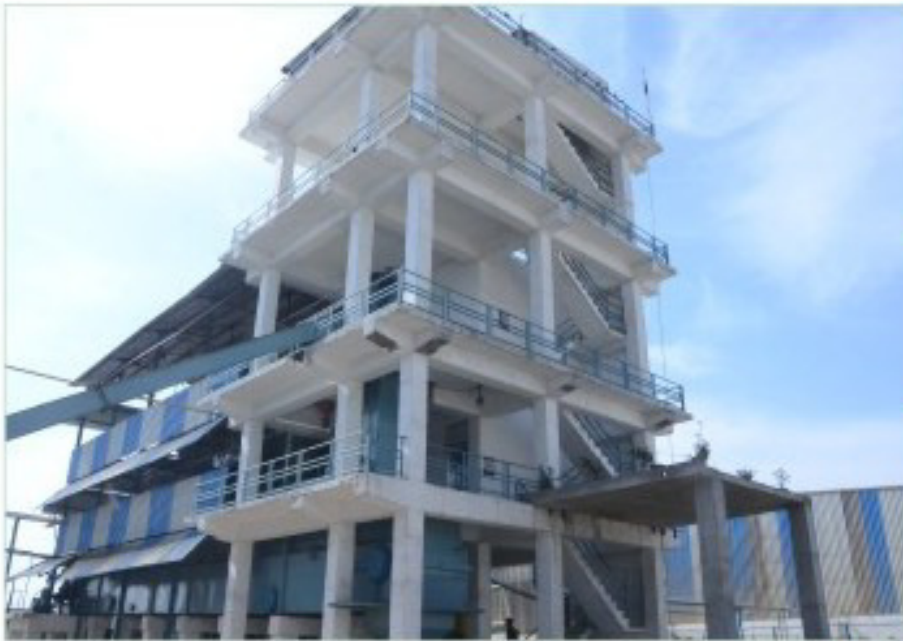
Solvent Extraction Plant Capacity 500 TPD,
