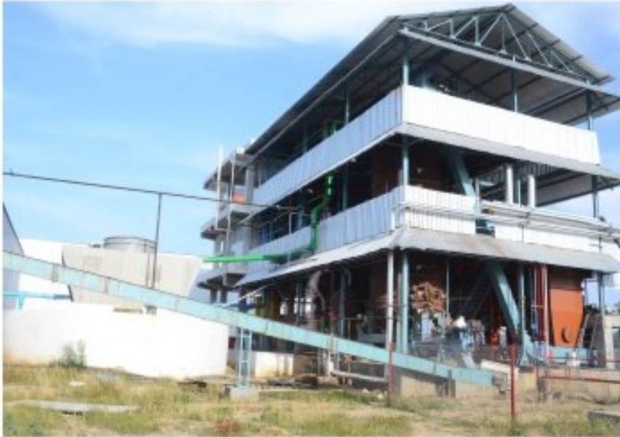
Solvent Extraction Plant Capacity 200 TPD,
