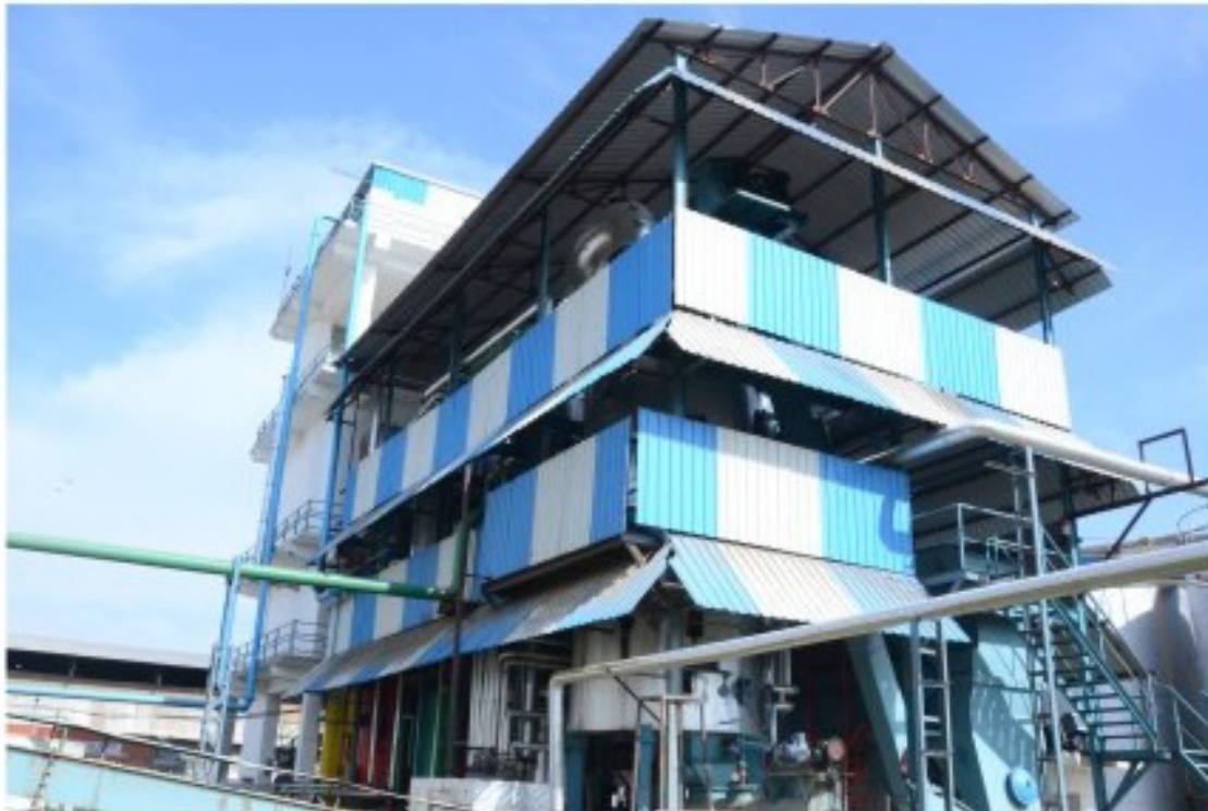
Solvent Extraction Plant Capacity 700 TPD
